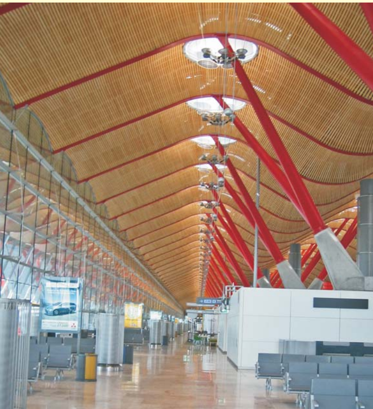
The glass curtain walls on Aeropuerto de Barajas are supported by high strength duplex 2205 and Type 316 stainless steel. (Figure 5). (Figure 5a below shows details) Photos courtesy: FOLCRÁ, Spain
