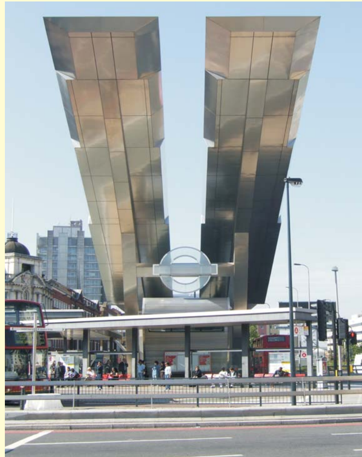
Vauxhall Cross Station, London (Figure 11) Photo credit: Thomas Pauly, Euro Inox
