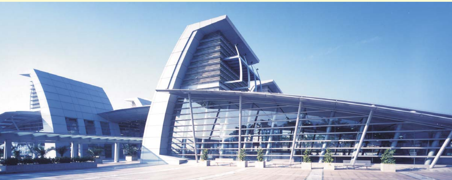
The high profile Type 316 stainless steel roof on Hong Kong's Kowloon Station is many visitors first introduction to the city. (Figure 4) Photo courtesy TFP Farrells
