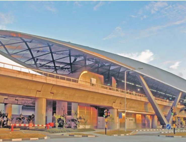
The spaceship inspired shapes of the domes on the Singapore Expo Center's MRT Station have titanium roofs and the sheltered areas and glass support system are Type 316 stainless steel. (Figure 9) Photo courtesy: Nickel Institute
