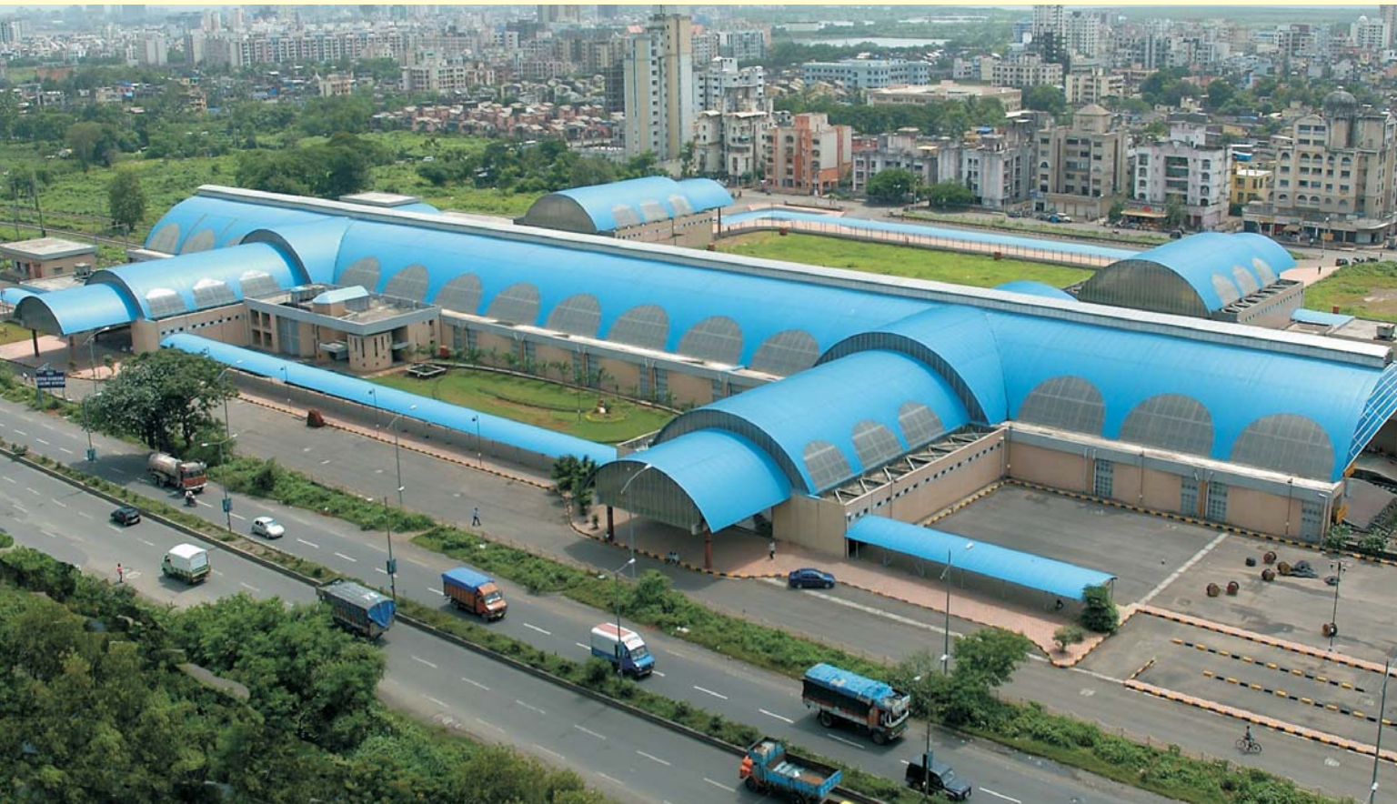
The Koperkhairane railway station at New Bombay used 10,000 square meters of painted Type 304 stainless for roofing Photo courtesy Salem Steel Plant (SAIL)
