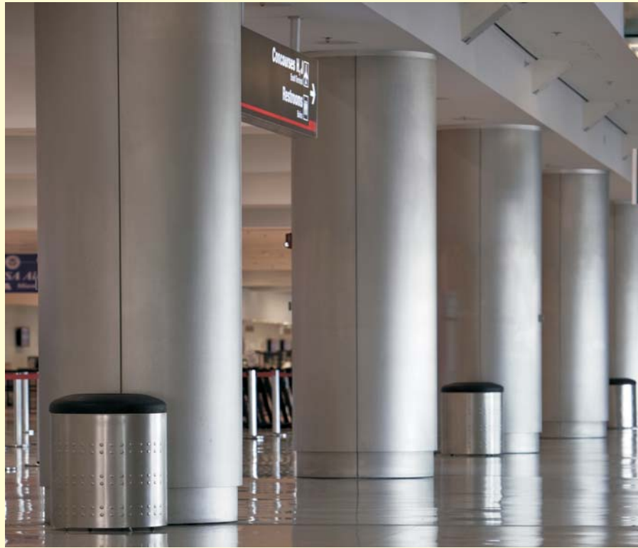
Columns clad in Type 304 stainless steel with bead blasted finish at Miami International (Figure 8a) Photo courtesy of Forms + Surfaces
