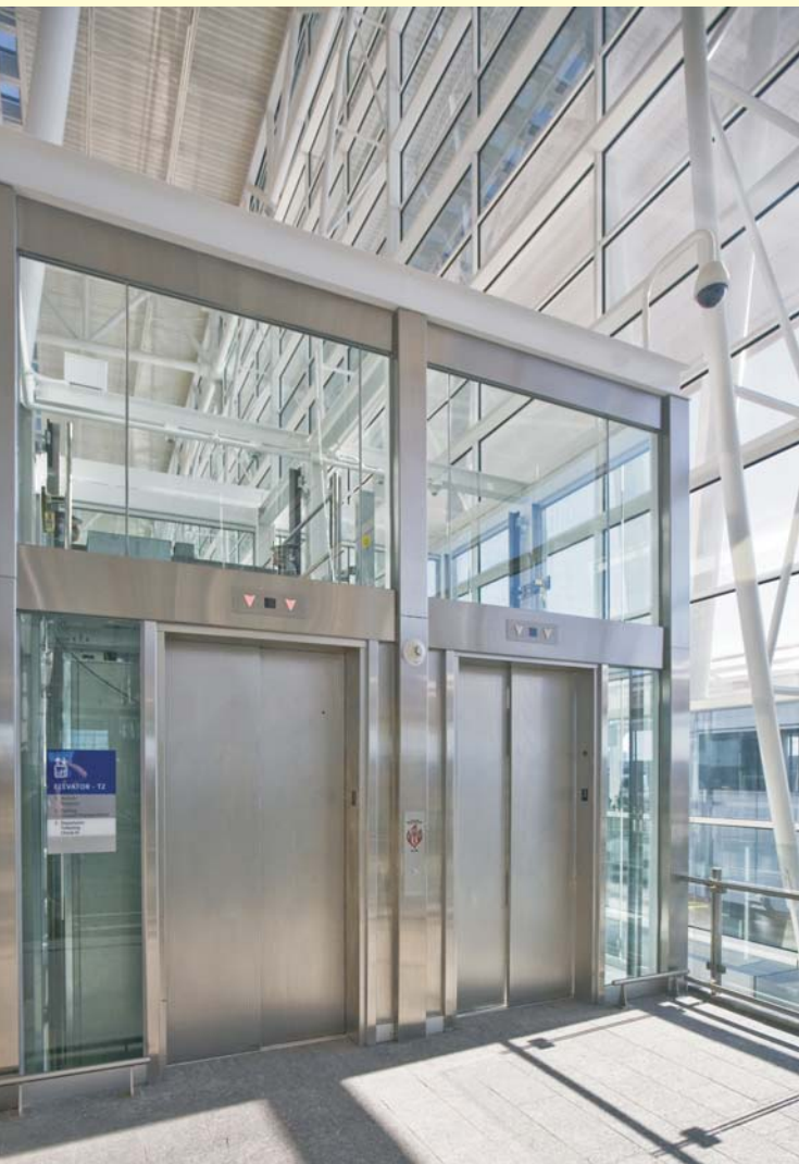
The new Colonel H. Weir Cook Terminal at Indianapolis International Airport used Type 304 stainless steel extensively in its interior. (Figure 7b) Photo courtesy of Forms + Surfaces
