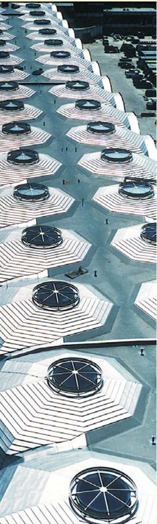
Roof of Ronald Reagan Airport (Figure 3) Photo courtesy Overly Manufacturing Co.,
