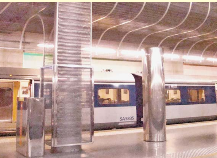
The interior of the new Britomart Train Station in Auckland New Zealand used woven Type 316 of the ceiling and column covers. Custom embossed and polished covers were used on the forced ventilation pillars around the tracks. (Figure 10) Photo courtesy: Nickel Institute, Catherine Houska photographer
