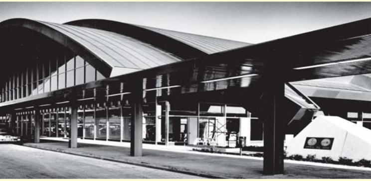
The stainless steel parabolic roof on the JFK International Arrivals Building (former Terminal 4, 1956). (Figure 1) Photo courtesy Overly Manufacturing Co.
