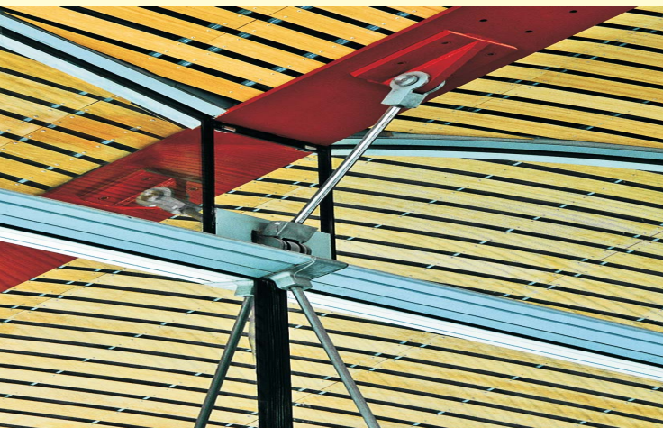
The glass curtain walls on Aeropuerto de Barajas are supported by high strength duplex 2205 and Type 316 stainless steel. (Figure 5). (Figure 5a below shows details) Photos courtesy: FOLCRÁ, Spain
